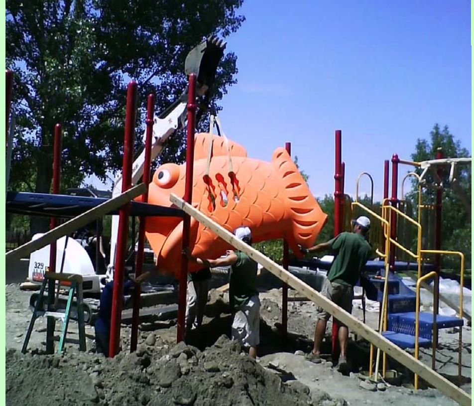
Centennial Park Installing New Play Structure
